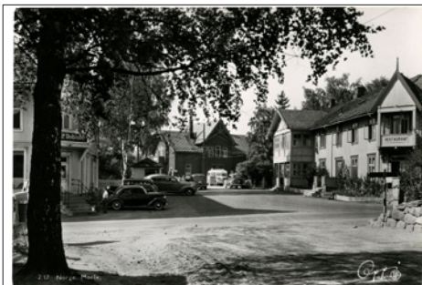
NR 385 IN Moelv, Oppi 217, ubr storf, kv 2
