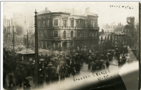
NR 77 HO Bergen Branden i Bergen Grand Hotel. K.Nyblin, ubr, kv 2-3 (liten Brett)
