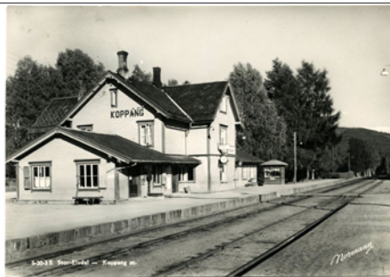
NR 378 HE Stor-Elvdal - Koppang st, Normann 5-20-35, stpl Koppang 43, kv 1
