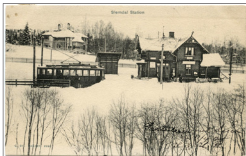
NR 401 OS Slemdal Station, C St 2297, br -06, kv 2 kr. 100
