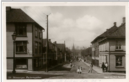
NR 415 RO Stavanger Pedersgaden, Johs. Floor 29, br.-22, kv 2
