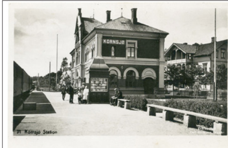
NR 173 ØF Kornsjø Station, Normann 71, stpl Kornsjø -30, kv 1-2
